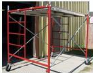
Scaffolding fully decked
