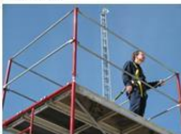
3 rd level with guardrails
