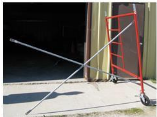
X-bracing attached to the first end frame
